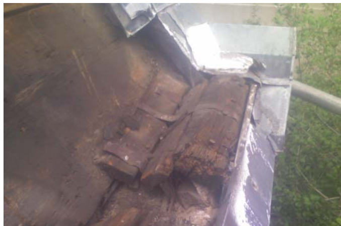
South East Altar Gutter Before
