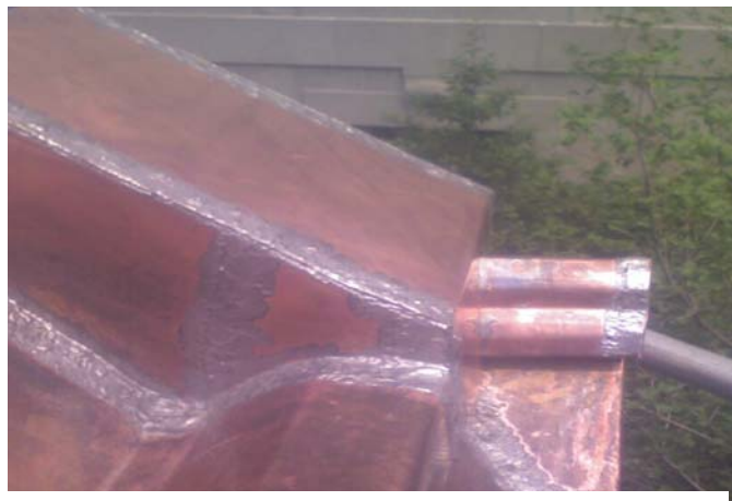
South East Altar Gutter After
